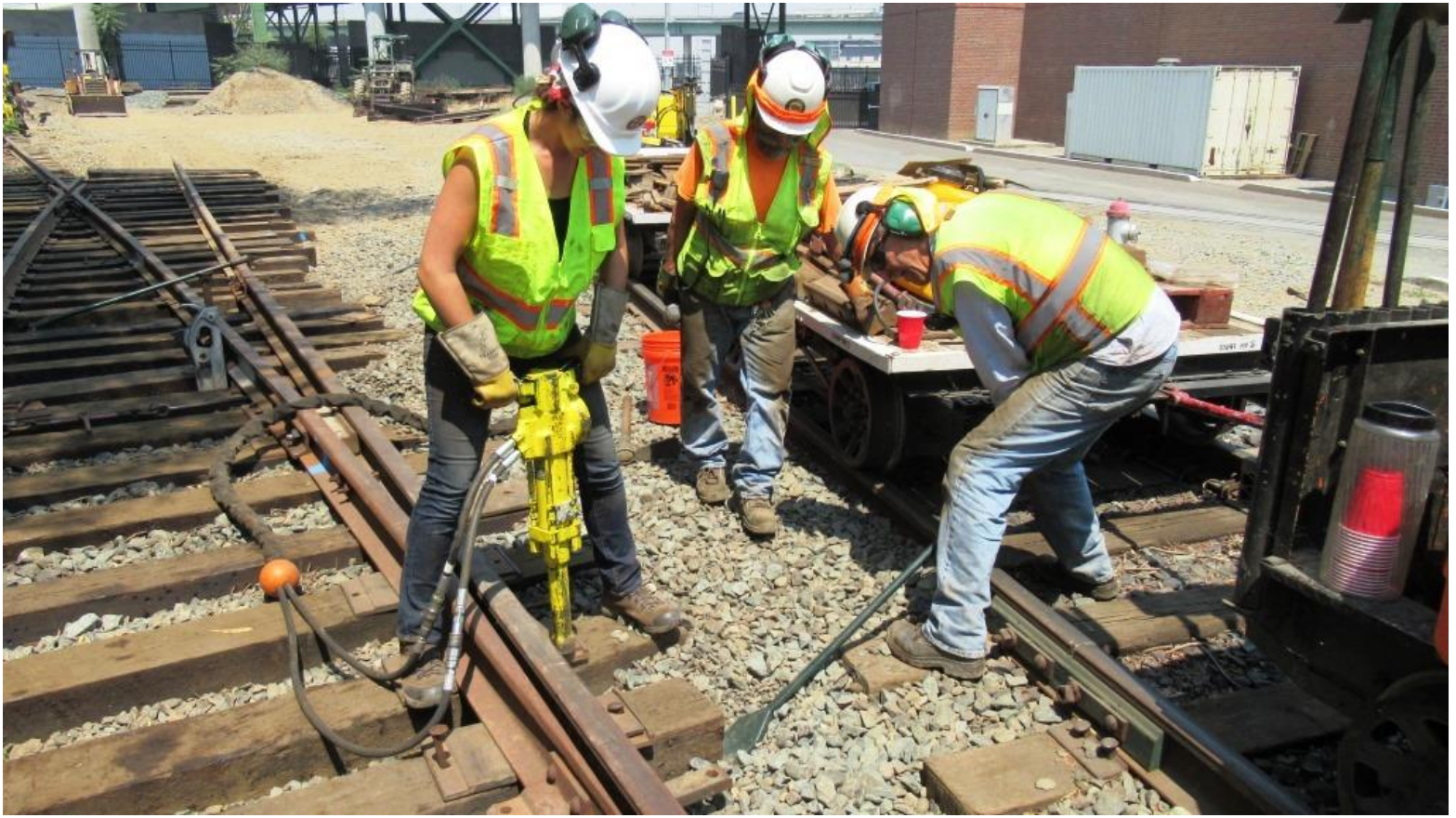
Steve nips the tie as Samantha gets some quality time with the hydraulic spike-driver
