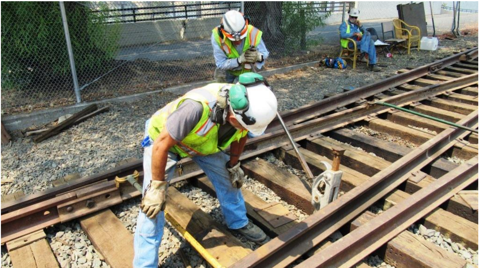
Steve and Ed use a track-jack to lift the rail sufficiently for inserting thick tie-plates
