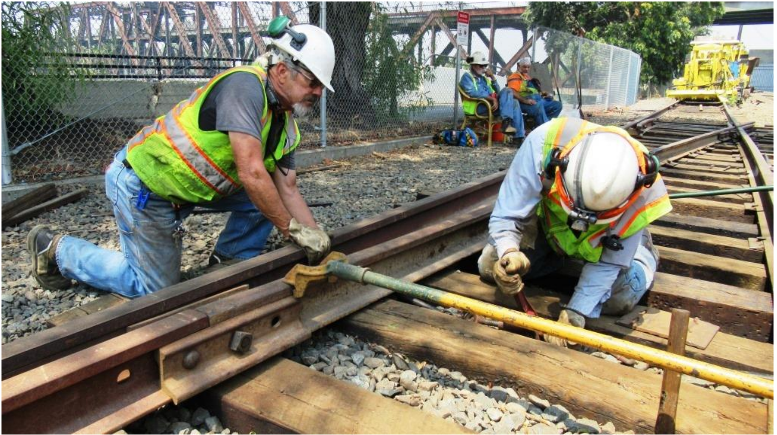
Ed and Steve use the grapple-gauger to pull the rails into gauge
