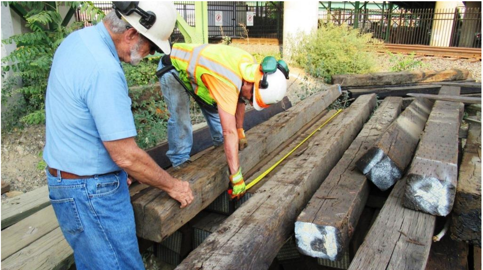
Alan and Joe search for a 10-foot tie in the extra-long tie pile
