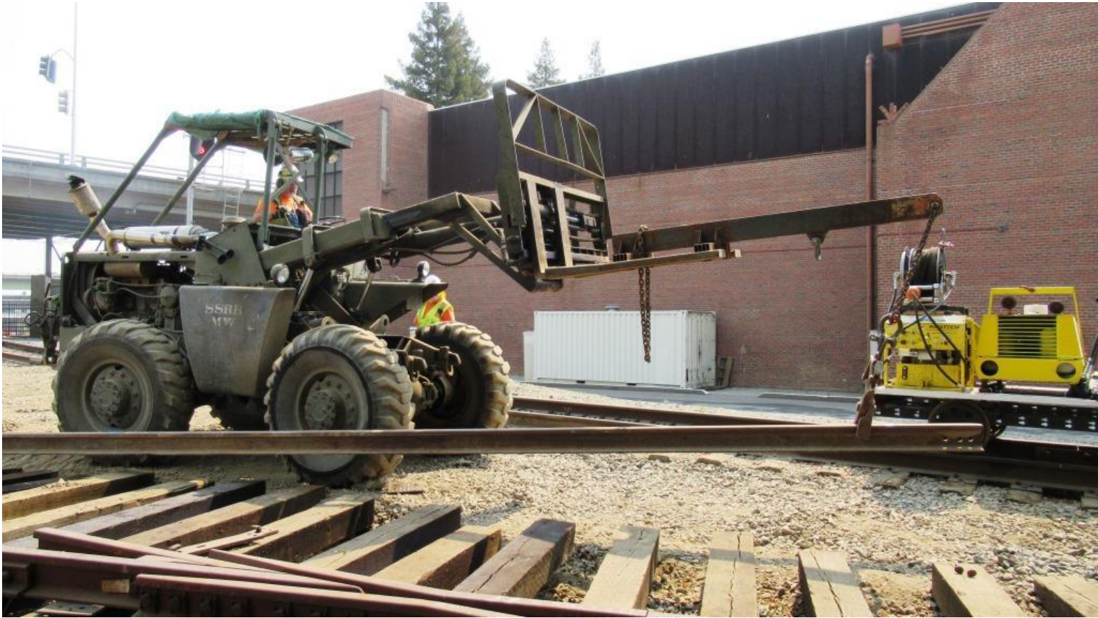
Mike F. on Big Green brings over a stick of rail for the diverging track
