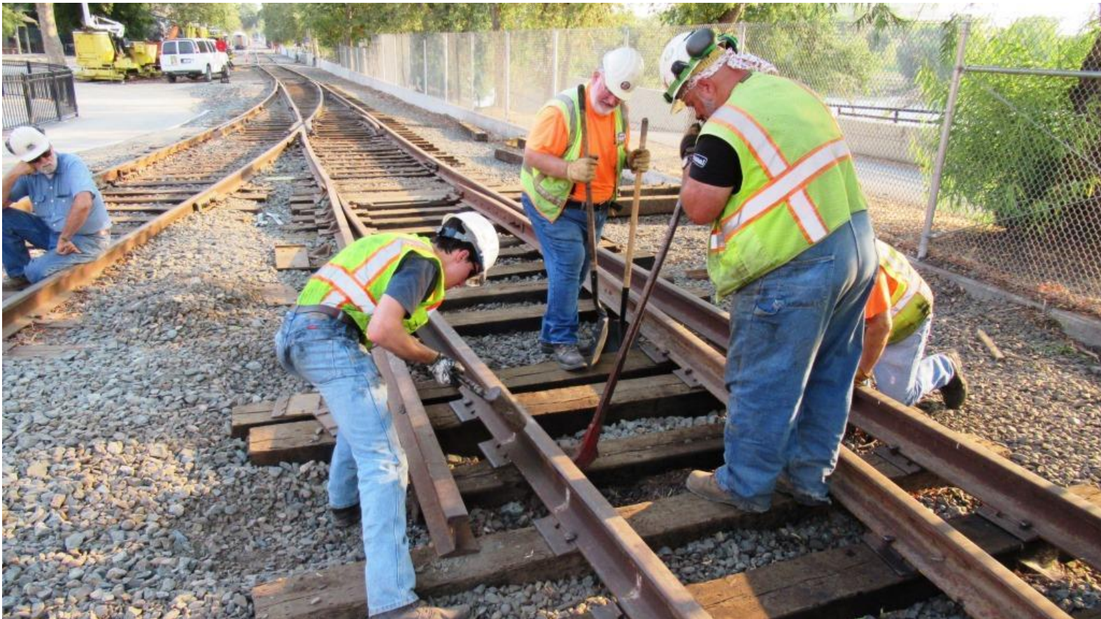
Mike F. nips the rail as Jack pounds out the tie-plate
