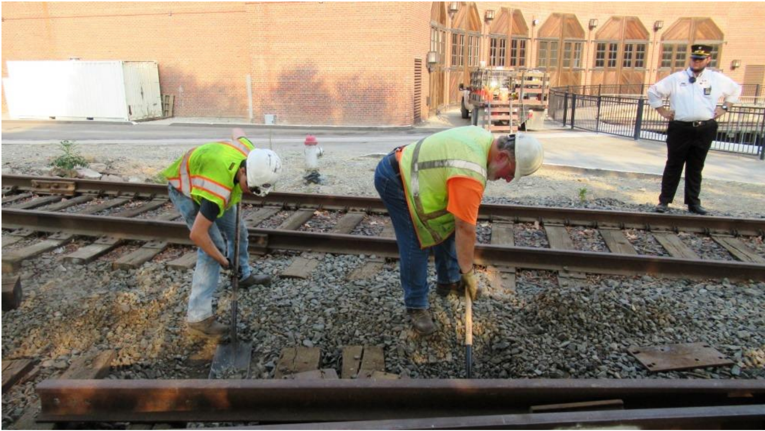
Jack and Frank dig out the ends of ties
