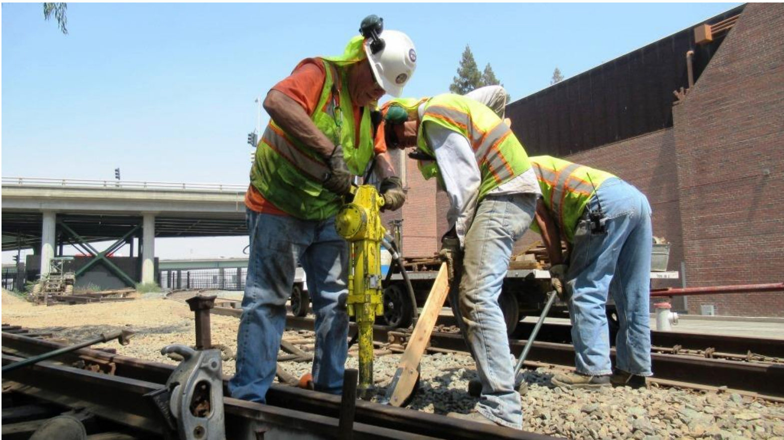
Steve uses the Steve Tool to hold the un-set spike in place as Bill drives it in
