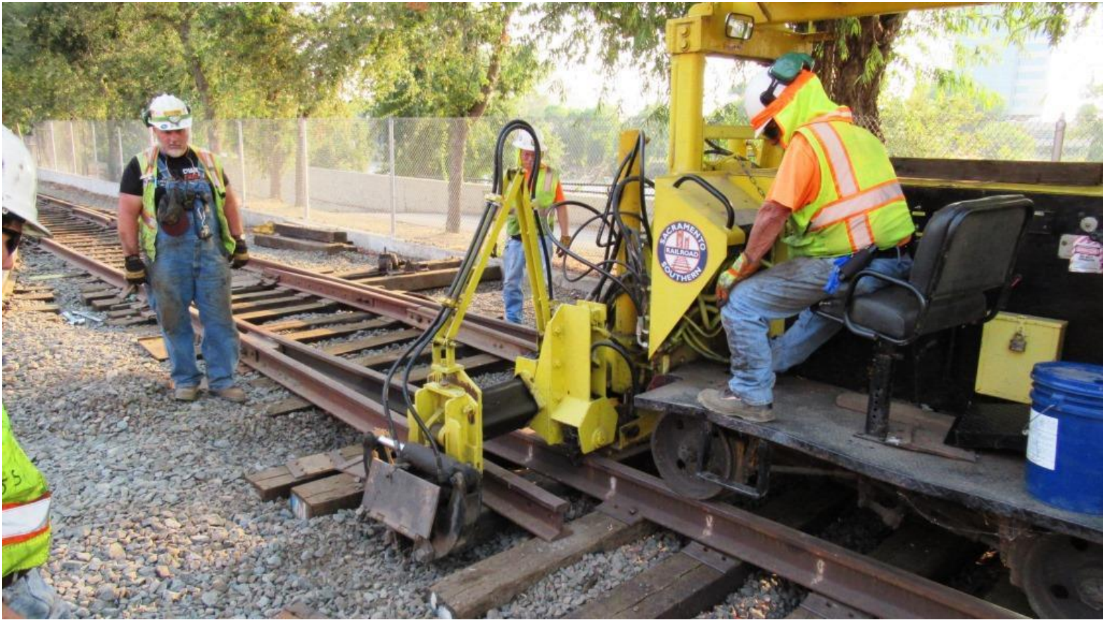
Joe brings in the Jackson 125 tie-exchanger, scoots the claws under the diverging rail, and gently grabs the very end of the tie being removed
