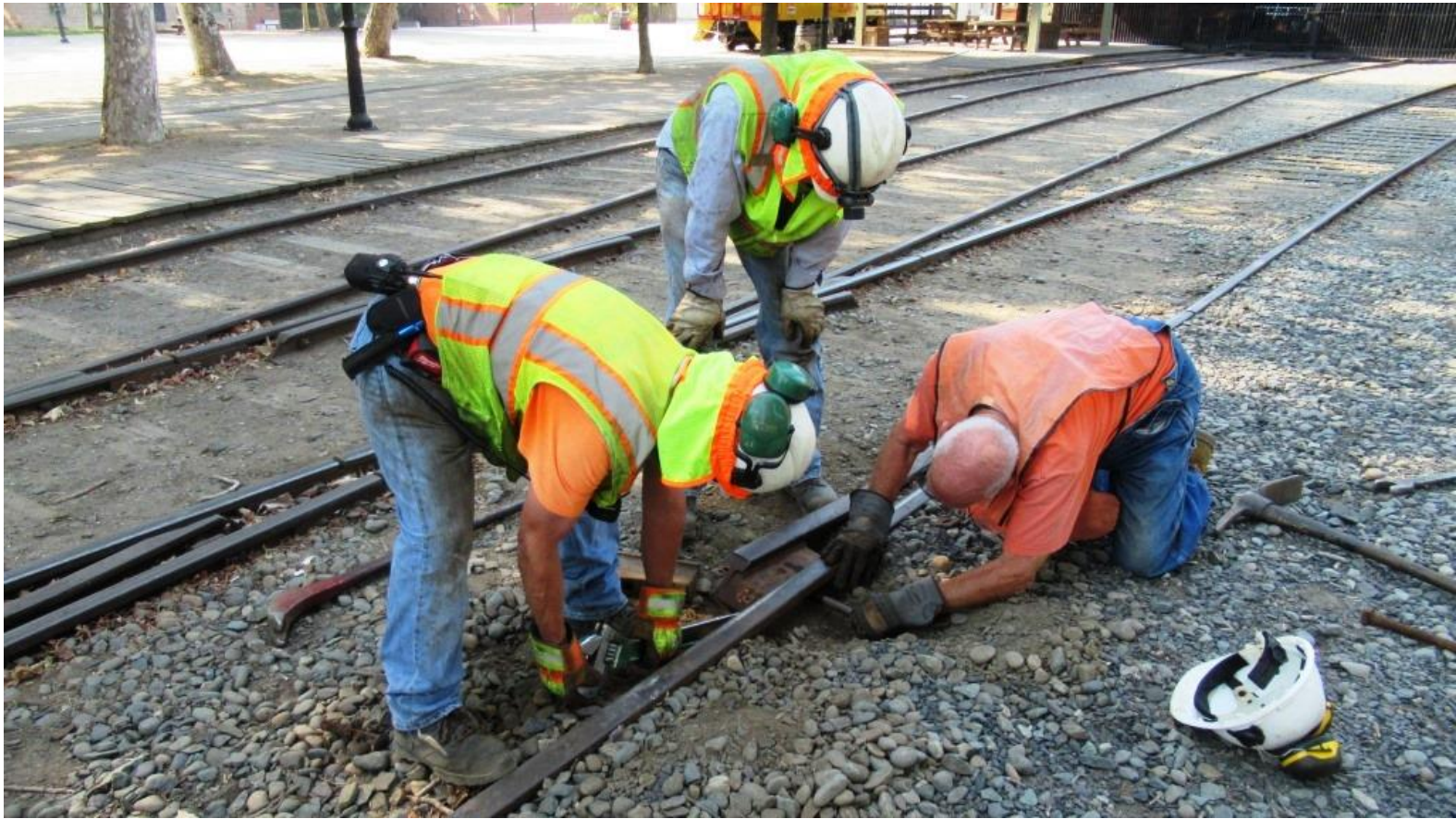
Joe, Steve, and Clem work feverishly to get the replacement block to fit with a stock-rail forged in 1891 and a guard-rail forged in 1903
