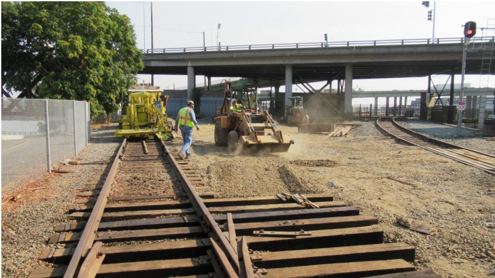
Ed gets the roadbed dug out for the placement of ties
