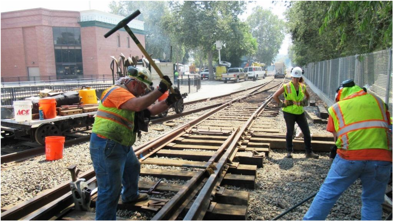
Bill nips the tie as Mike F. drives spikes the old-fashioned way
