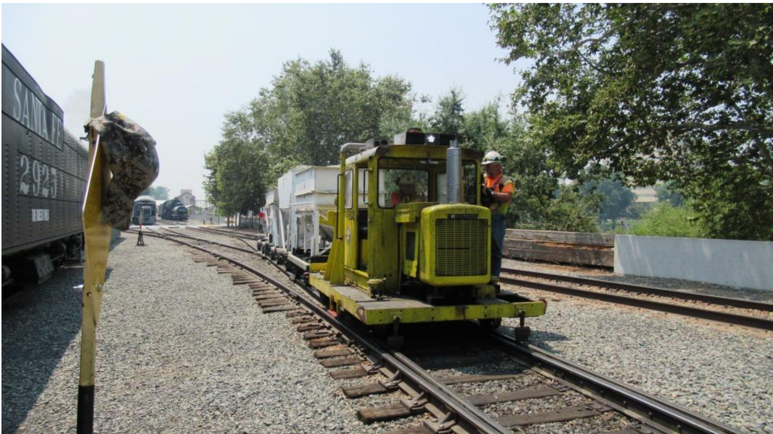
Bill and Mike F. bring the Kalamazoo pulling heavy hoppers to roll over the new guard-rail assembly to help settle the track
