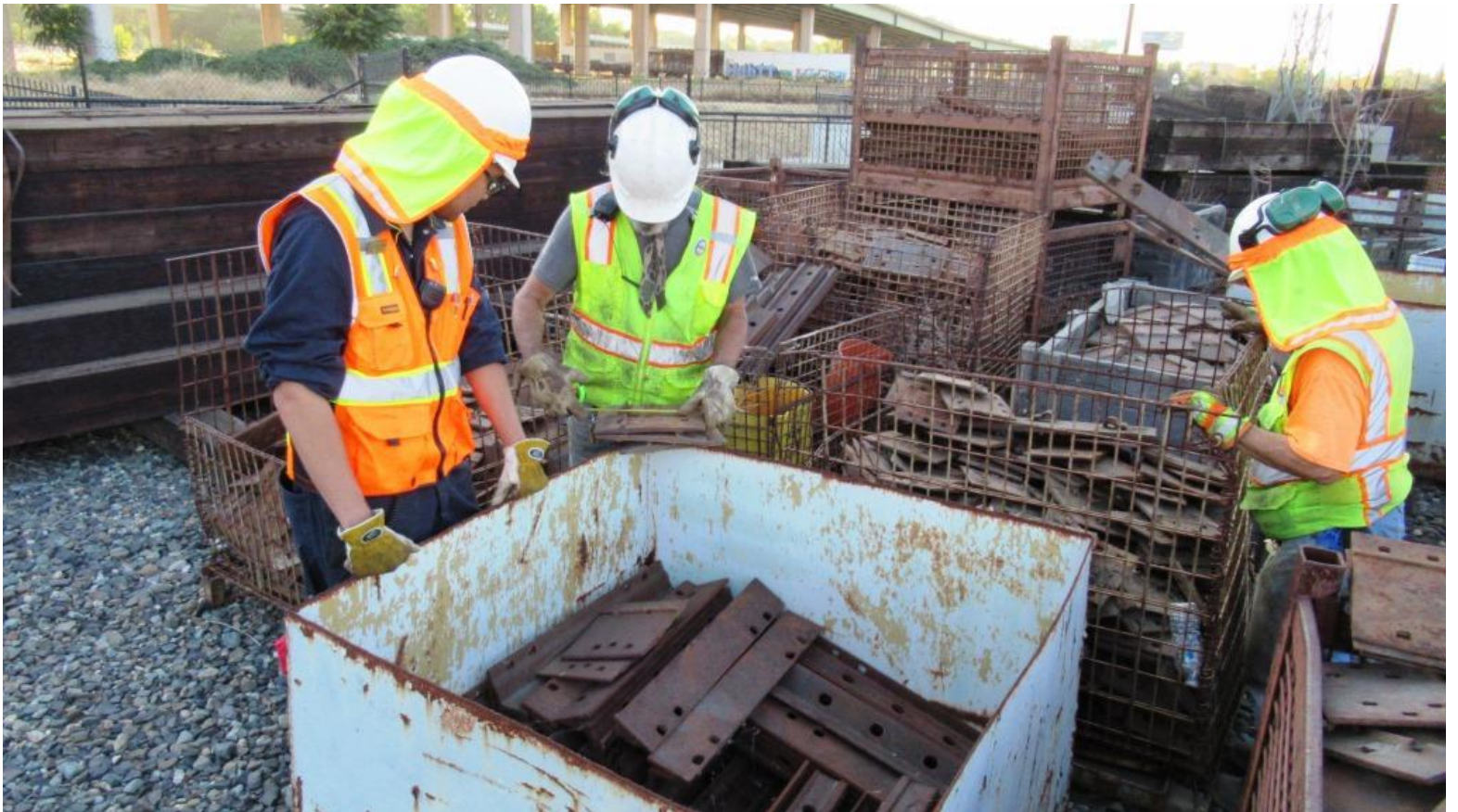
Ed show Kyle how to determine if it's the right sized plate by measuring the distance between the spike-holes
