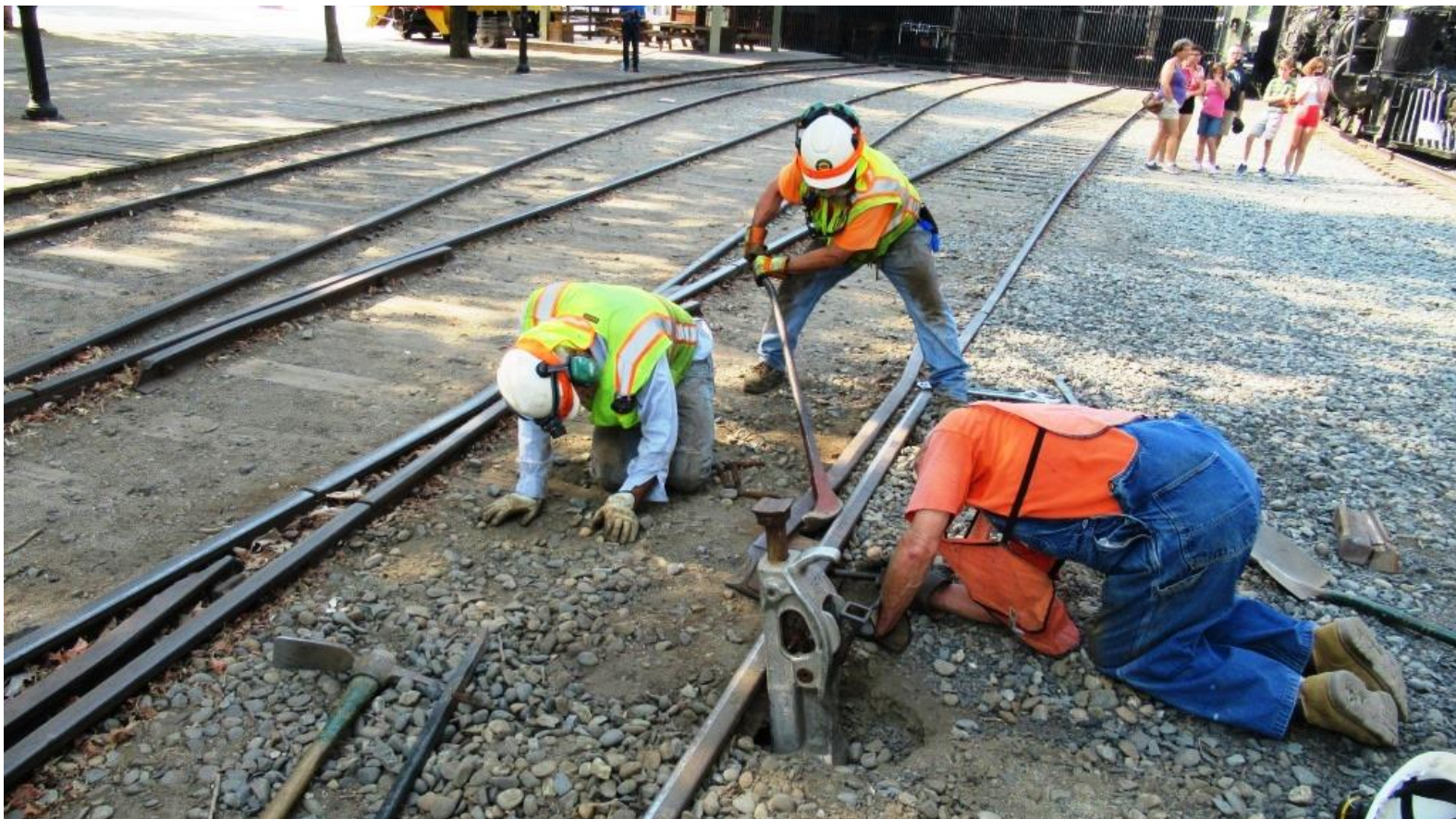
Pushing, pulling, lifting, lowering, Steve, Joe, and Clem continue their quest to make it fit – or else!
