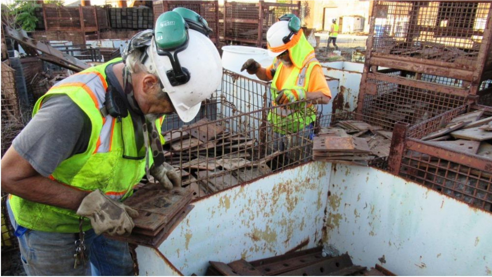
Ed and Joe search out tie-plates for the 110-pound rail of the diverging track
