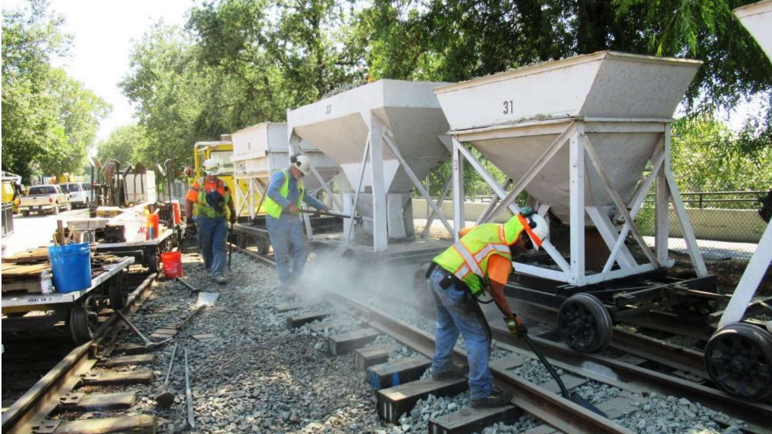
Alan now drops rock from the center-dump ballast hopper
