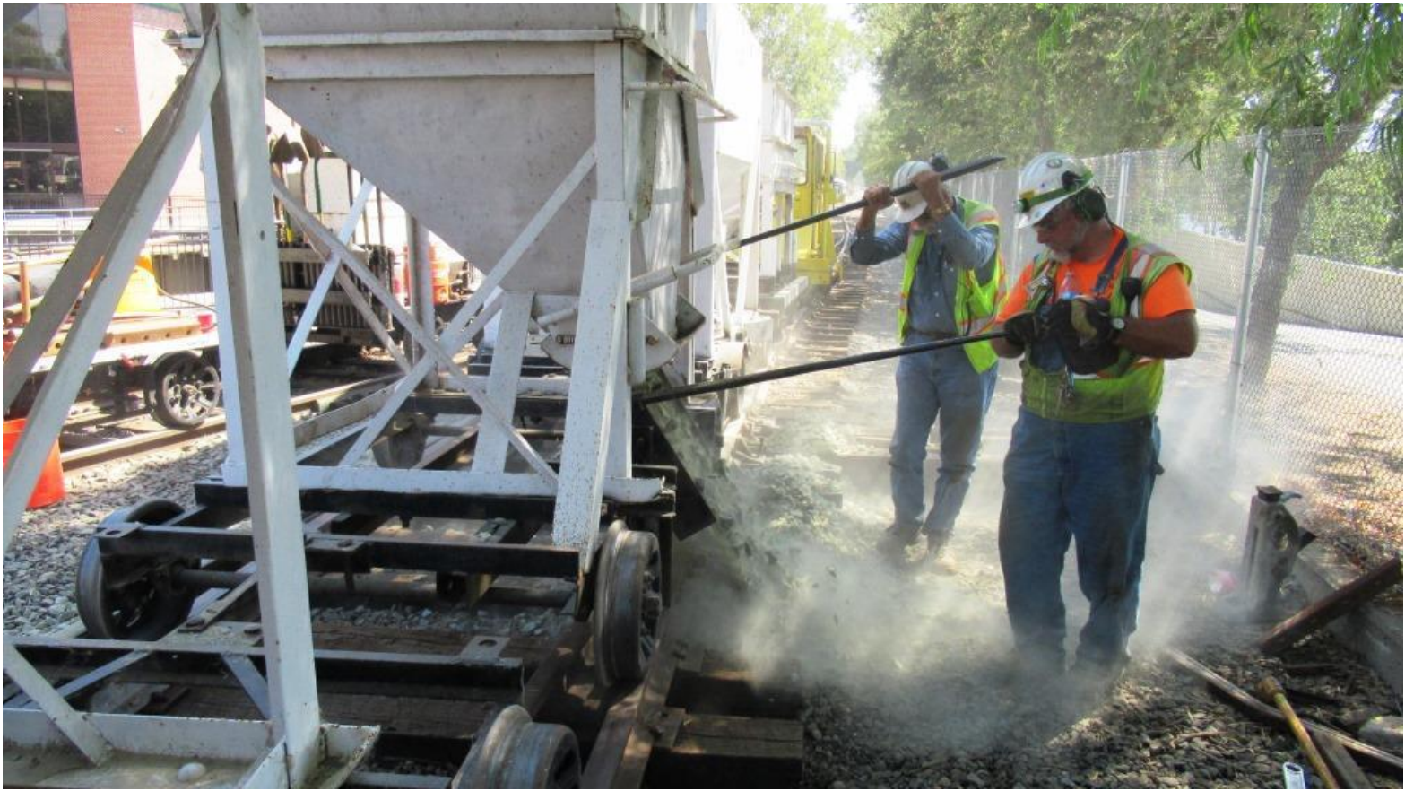
Bring in the hoppers! Alan and Mike F. regulate the flow of rock from the hoppers as ballasting of the switch begins
