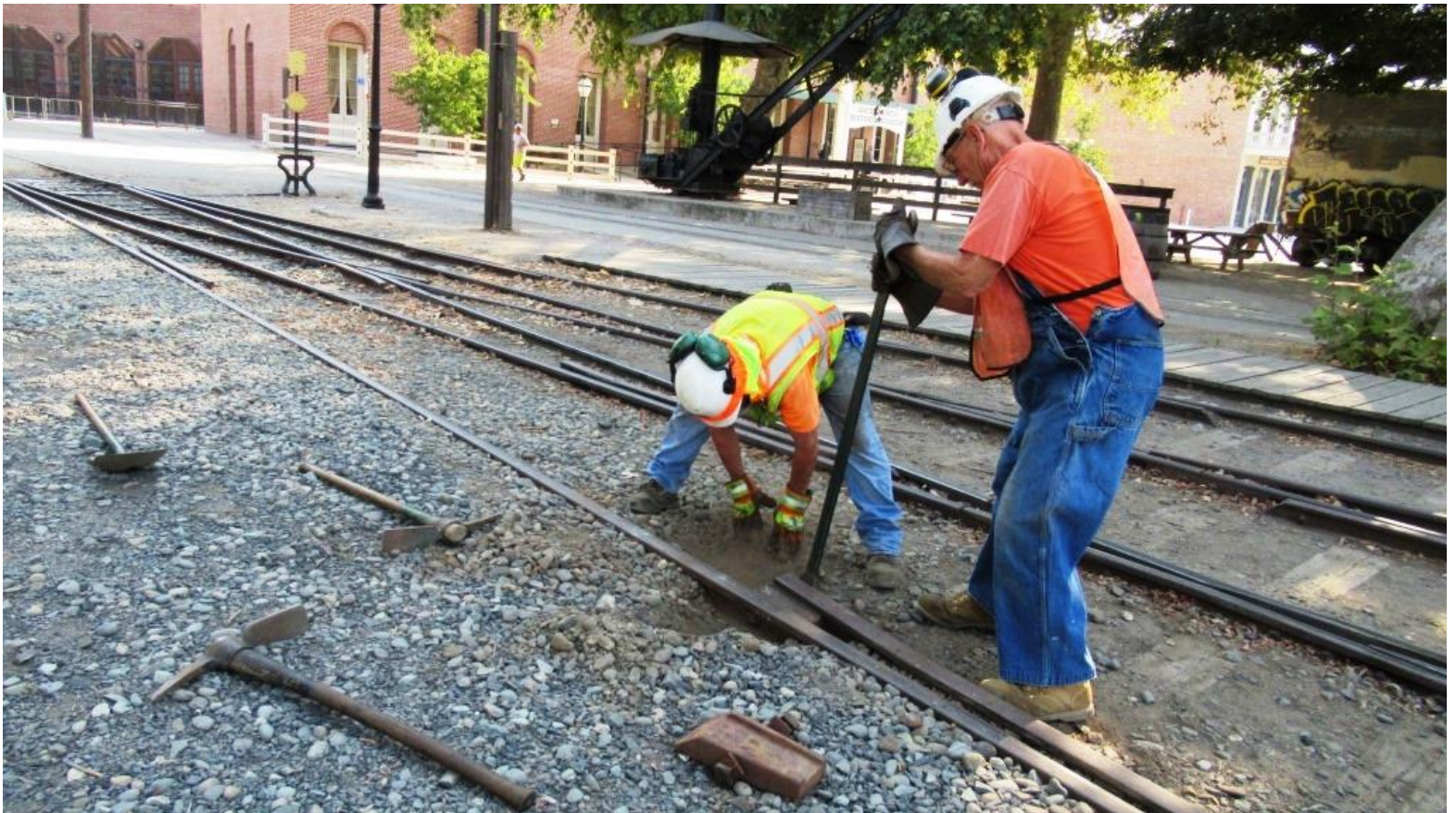
Joe and Clem get started removing the busted guard-rail block
