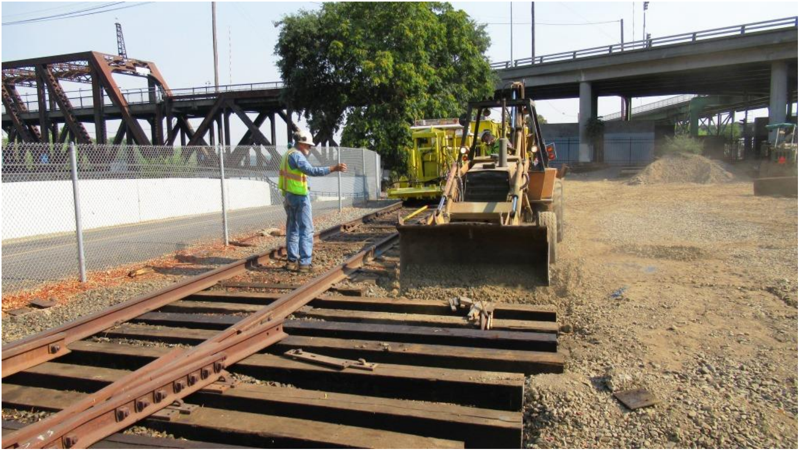
Meanwhile, up on the hill, Alan give Ed some guidance on grading the roadbed for the diverging track
